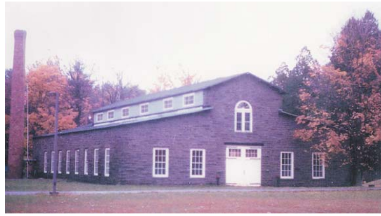
Edmund T. Cloonan Water Treatment Plant
